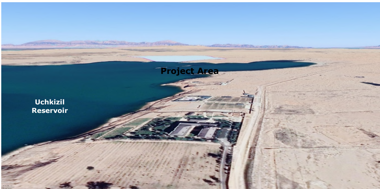
Figure 112: View of the Project Area from the south direction
